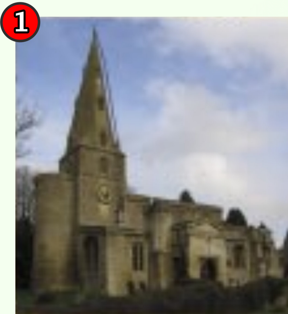
1 ST. ANDREWS CHURCH has an unusual Saxon stair turret dating from 750 to 800 A.D. An earlier church was burned down during the 9th Century Danish invasions. To the right of the path leading to the church is the Lyvedon family vault and inside the church is the tomb of Lord Lyvedon.
