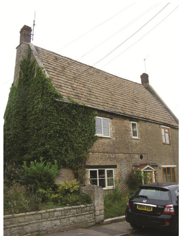
Nos.22 – 24 Bridge Street
