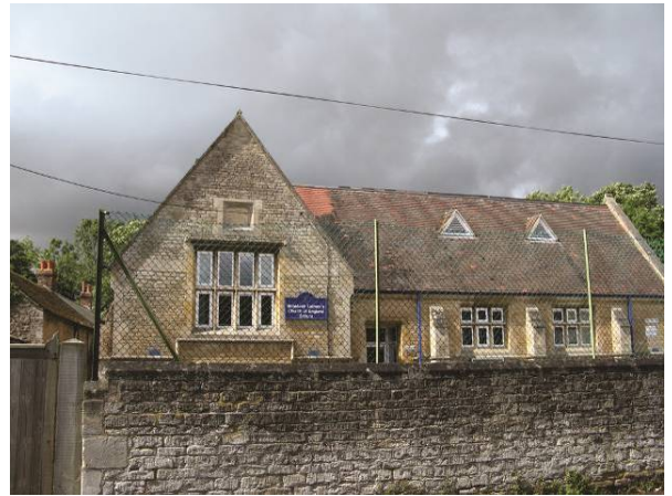
Latham's School, Latham Street
