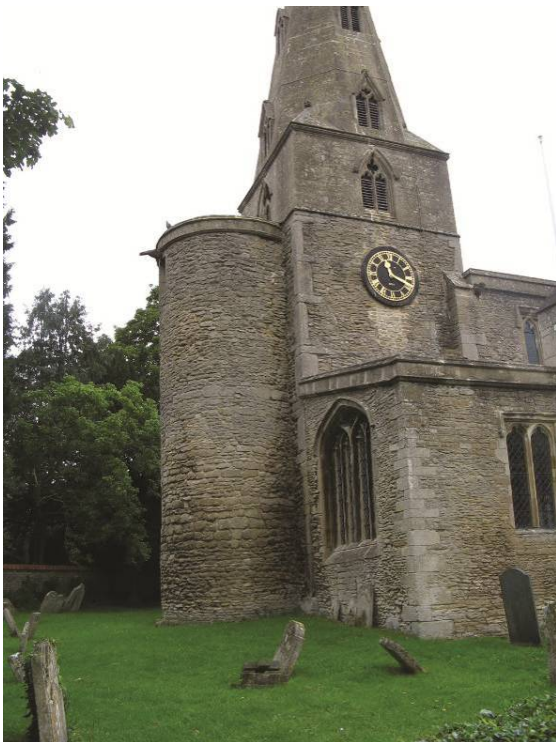
The late 10 th century staircase, St Andrew's Church
