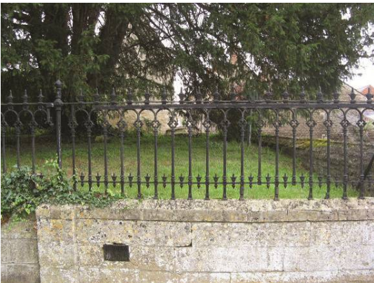
Cast iron railings to St Andrew's Churchyard
