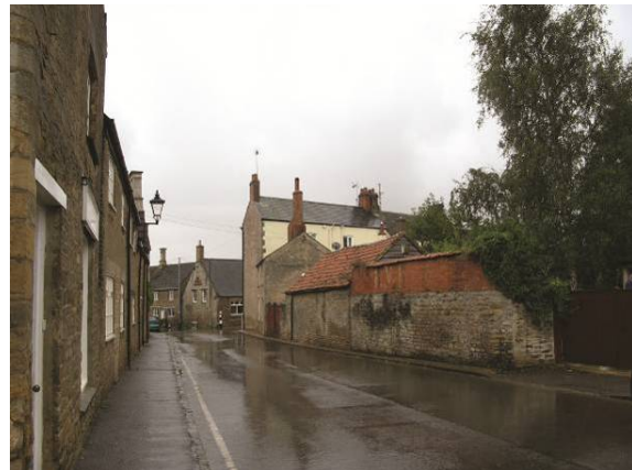
Raised wall in brick at rear of No.2 Hall Hill
