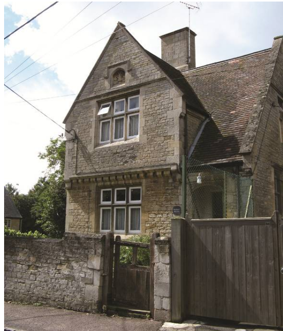
Headmaster's House, Brigstock and Lathams C of E Primary School, Latham Street
