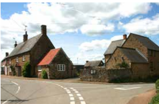
Variations in setting and level of the roofline
