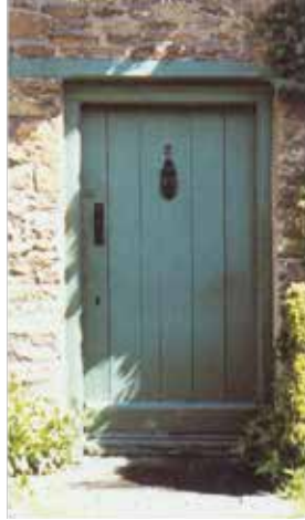
Vertical boarded, ledged and braced door
