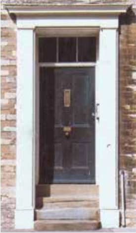
Four-panelled door under fanlight
