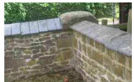
Capped with blue brick
