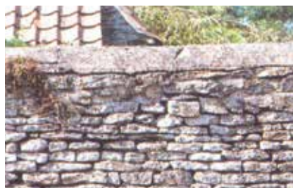
Capped with mortar
