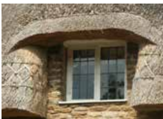
Swept dormer in long straw thatch
