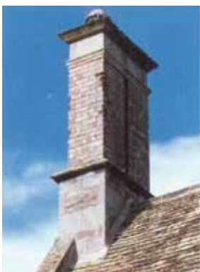
Brick and dressed stone stack on the ridge line
