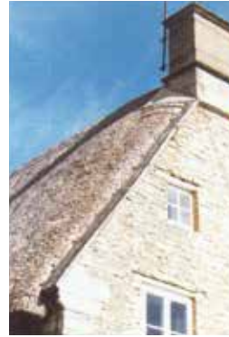
Coped Gable parapet with kneeler stone
