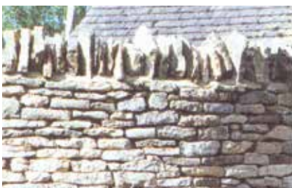
Capped with stone
