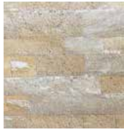
Ashlar with regular coursing and fine joints
