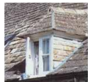
Hipped dormer on Collyweston roof
