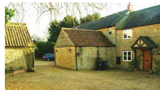
Garages well-integrated in this 20th C conversion using a mixture of traditional materials.
