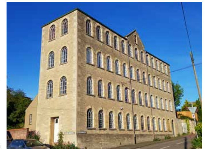
Figure 15: Wallis's Mill Photo: Bobsky
