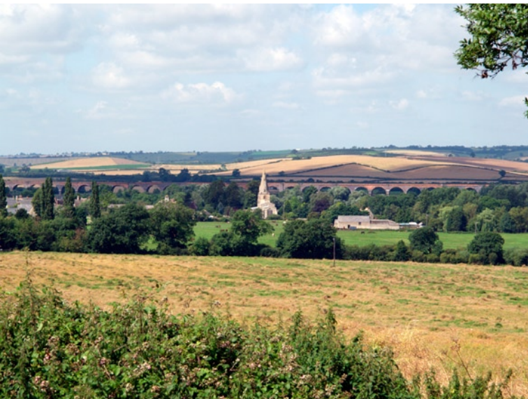
Harringworth Viaduct as a backdrop to the village and church
