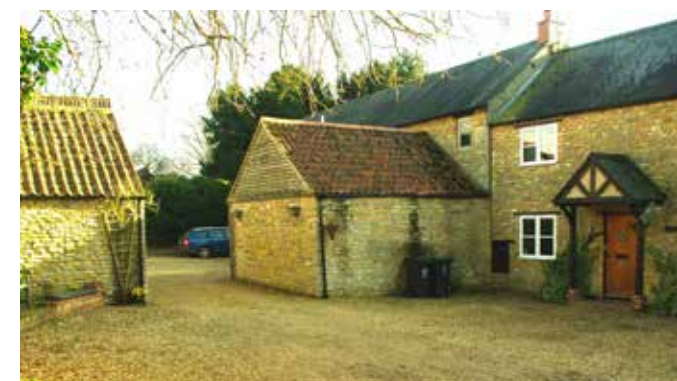
Garages well-integrated in this 20th C conversion using a mixture of traditional materials.
