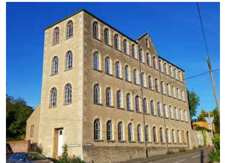
Figure 15: Wallis's Mill Photo: Bobsky
