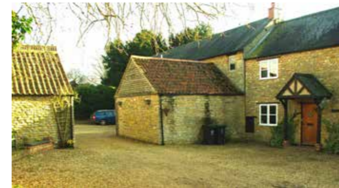
Garages well-integrated in this 20th C conversion using a mixture of traditional materials.
