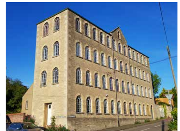
Figure 15: Wallis's Mill Photo: Bobsky
