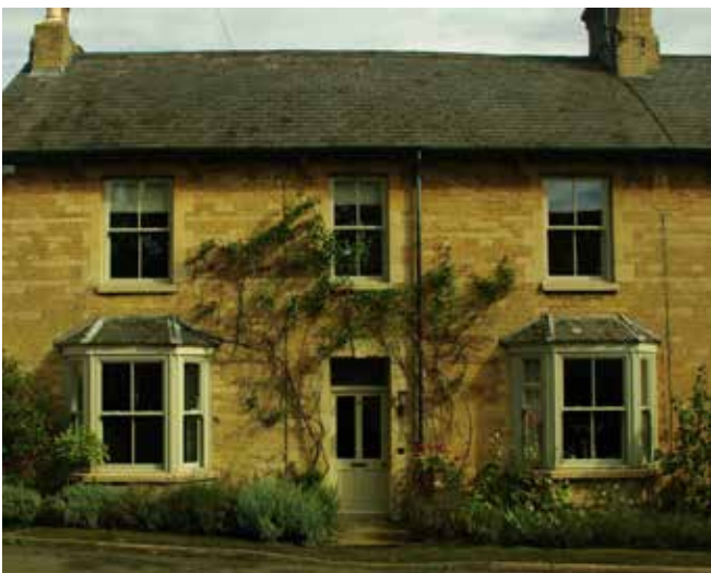
Carefully chosen replacement windows match the period of the house.
